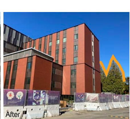
The BHTF with three western redcedars behind the building (outlined). Photo from October 2023.
